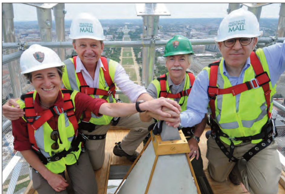
Interior Secretary Sally Jewell, along with John "Chip" Akridge, National Park Service Director Jon Jarvis and David Rubenstein touch the top of the Washington Monument. The Washington Monument is currently covered in scaffolding for repairs from an August 2011 earthquake. Photo: Tami A. Hellemann
